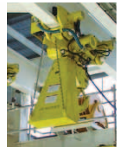
BOP chain hoist
